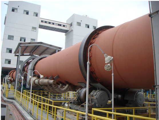
Cement kiln: 1450 °C
